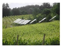
same area of land for both solar voltaic power as well as for agriculture. The coexistence of solar panels and crops implies a sharing of light and land between these two types of production.
